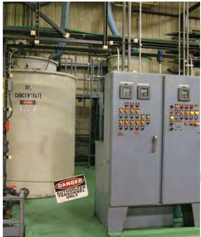
Above: Removing oil: the first stage of water recycling at the HiTech division of New Hampshire Ball Bearing.
